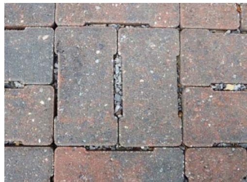
(1) Looking uphill, the Admission parking lot. (2) Close-up of the permeable brick showing gravel underneath.
